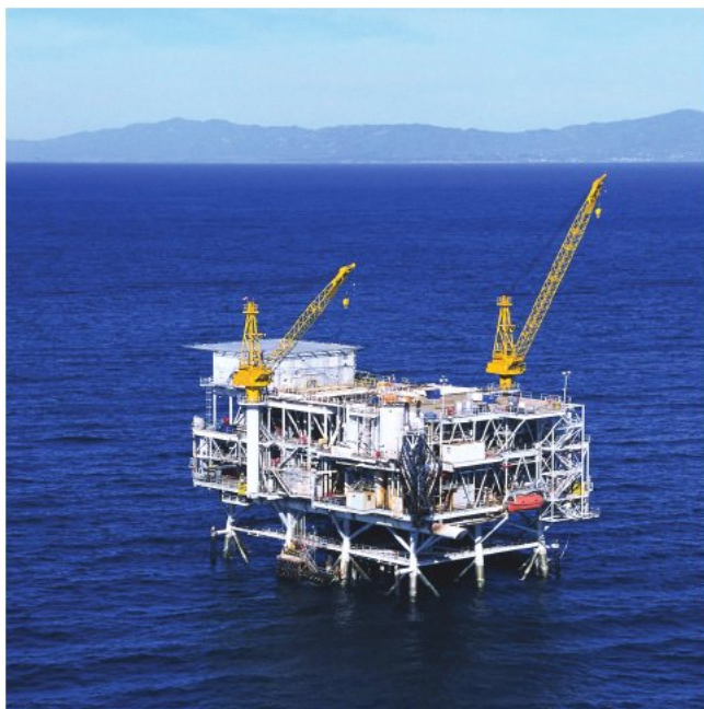
FIGURE 4.23 Offshore oil drilling platform. Constructed on tall stilts, drilling platforms are important for extracting petroleum reserves from beneath the continental shelves.
