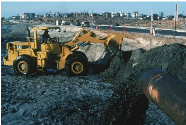
FIGURE 10.26 Beach replenishment. Beach replenishment projects, such as this one in Carlsbad, California, are used to widen beaches. Beach replenishment involves dredging sand from offshore or coastal locations, pumping it through a pipe ( lower right ), and spreading it across the beach.
