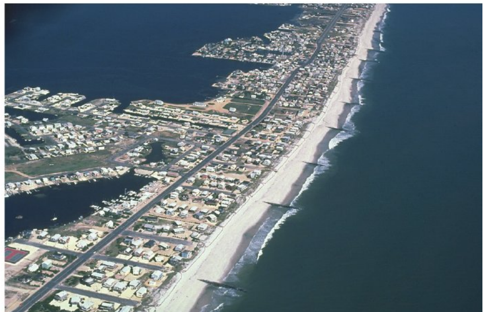
FIGURE 10.19 Groin field. A series of groins has been built along the shoreline north of Ship Bottom, New Jersey, in an attempt to trap sand, altering the distribution of sand on the beach. The view is toward the north, and the primary direction of longshore current is toward the bottom of the photo (toward the south).
