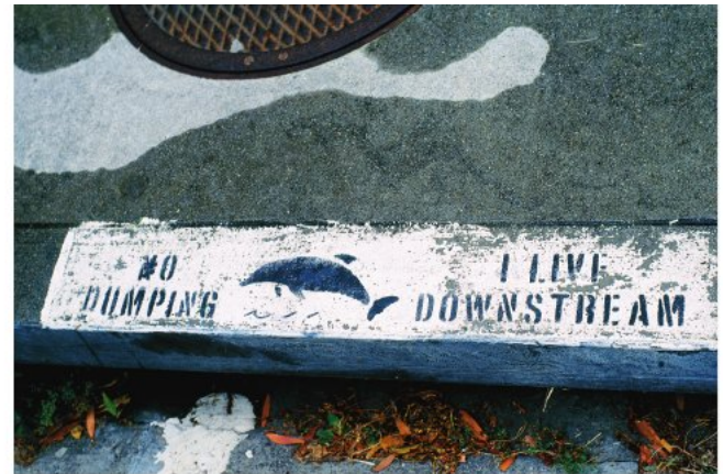
FIGURE 11.27 A labeled storm drain that leads to the ocean. Although many people believe that storm drain runoff is processed by sewage treatment plants, any material that enters storm drains goes directly into streams or the ocean.
