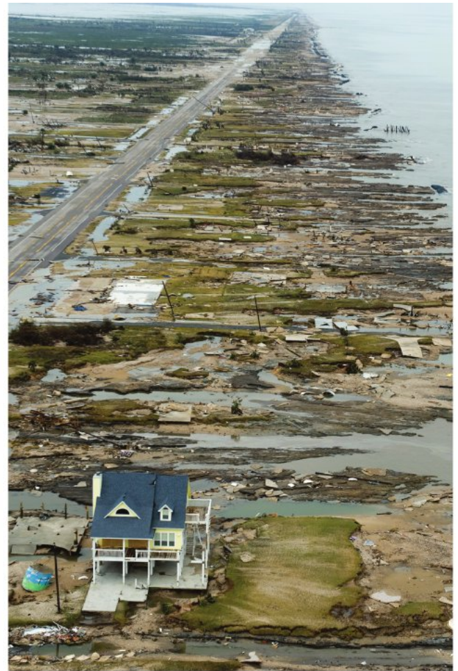
FIGURE 6.21 Damage from Hurricane Ike in 2008. Hurricane Ike, which made landfall in Gilchrist, Texas, was the third most destructive hurricane to ever make landfall in the United States.
